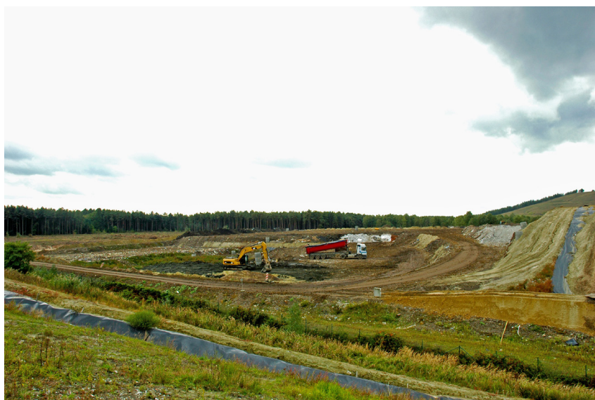
ELFM excavation at the Remo landfill site in Belgium, where the benchmark Closing the Circle ELFM project is developed
